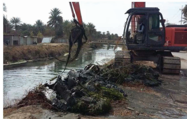
Fig. 1. Dredging process on AlMahawil stream
